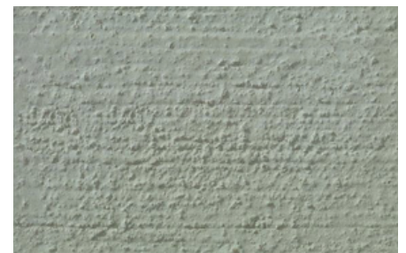
GREEN INTEGRAL COLORED CONCRETE (ADDED COST)
